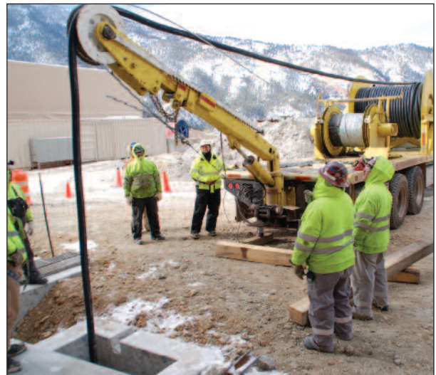
970' vertical single-messenger MPF borehole installation.
